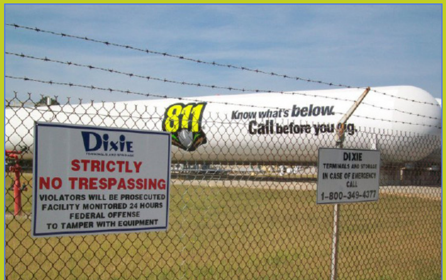
Dixie Pipeline's tanks in Lexington along Highway 1.
